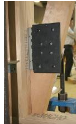
Picture 3: New brace fastener installed at the end of brace
