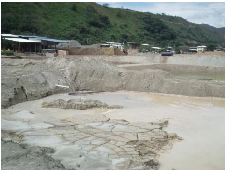
Figure 22. Tailings ponds to collect mercury-containing tailings mixed with other type of metallurgical residues.
