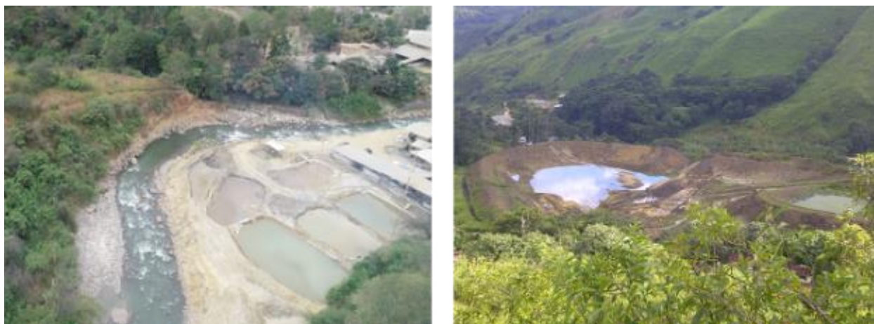
Figure 23. Tailings pond located next to the waterside and in a narrow terrain of an ASGM mining community (left picture). The topography of the area has some implications in selecting the site for large quantities of tailings disposal (right picture). The following problems can be anticipated: a) The walls of the tailings' storage consist of mine tailings. b) The containment wall is too close to the river with an enormous risk of contamination by liquefaction. c) There is a high risk of containment failure by an overflow of the river or a break due to high rainfall. Another important issue is the seepage and leakage through the bottom of the pond, dust emissions, and direct exposure of the nearby communities.
